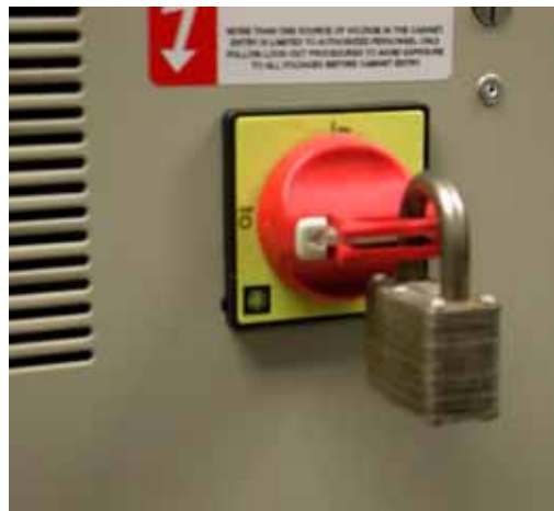
Fig 1.6 Disconnect Handle Positions – Shown OFF, With Padlock
