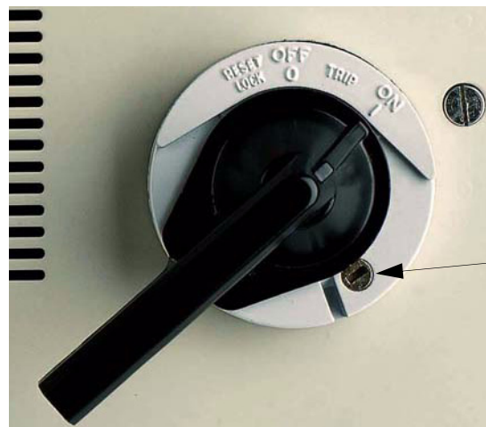
Fig 1.5 MCP Handle Positions – RESET/LOCK, OFF, TRIP, ON Shown in the “ON” position
