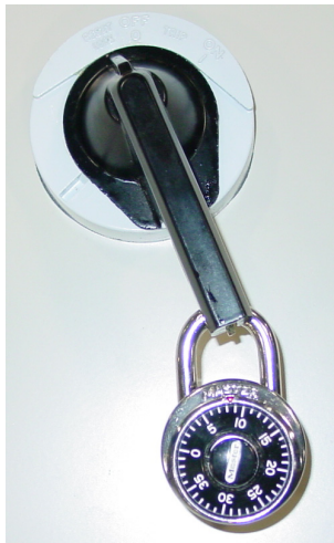
Fig 1.6 MCP Handle Positions – Shown OFF, With Padlock
