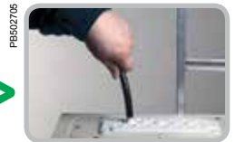
Pull the cable or tube back some 20 mm to lock it.
