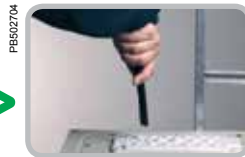
Push the cable or tube through the guide hole.
