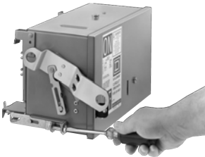
Figure 112 - Interlock Example
