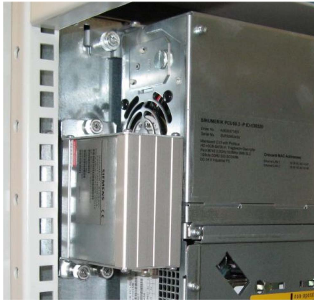
Figure 12-15 Direct key module after installation
