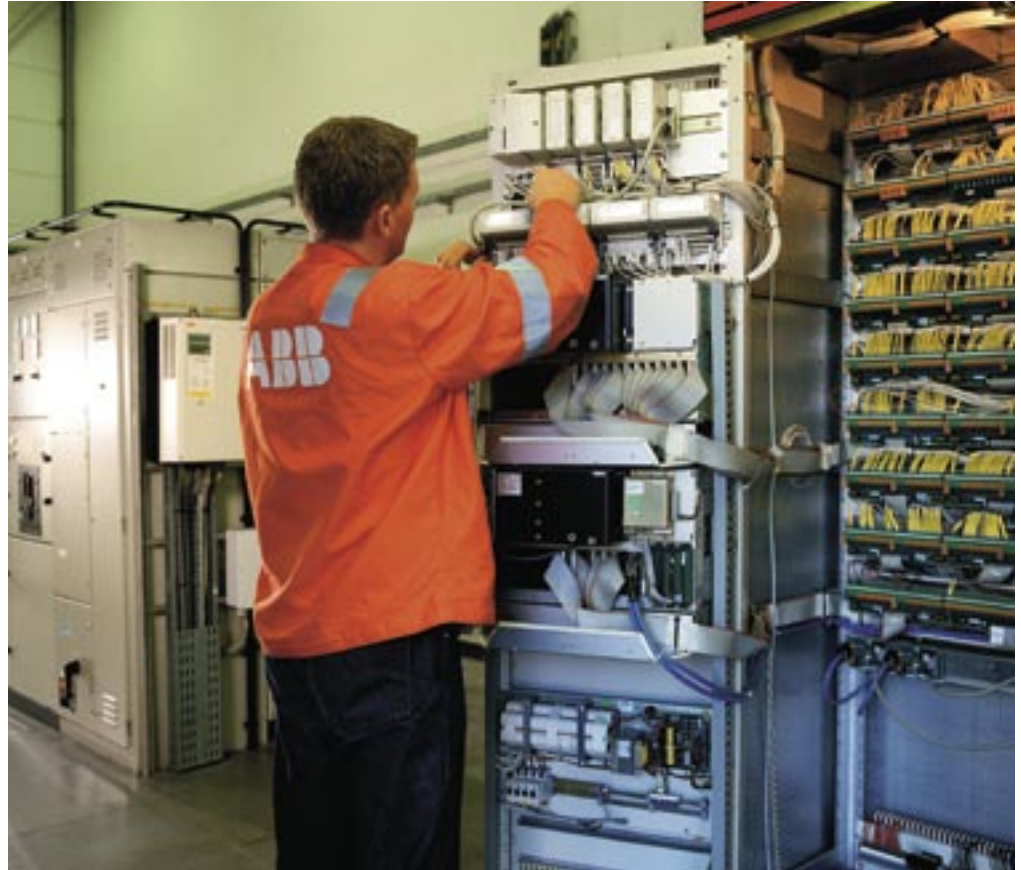
Figure 6. 800xA Control and /IO makes connected field devices transparently available to applications and people, for everything from device configuration and setup to production monitoring and maintenance.
