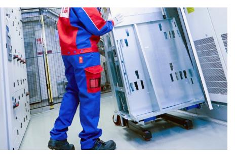
Drive modules are heavy objects with a high center of gravity, so moving them can cause a risk of tipping over. However, moving these modules is a necessary part of the installation and maintenance process during the lifetime of the drive. ABB offers different tools to ensure that moving the modules becomes easier and safer for service personnel.
