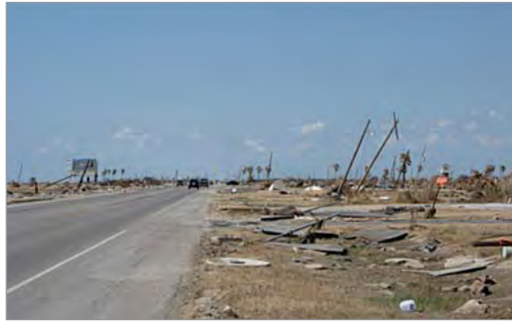
Figure A4-1 – Gilchrist, Texas, after Hurricane Ike [24]
