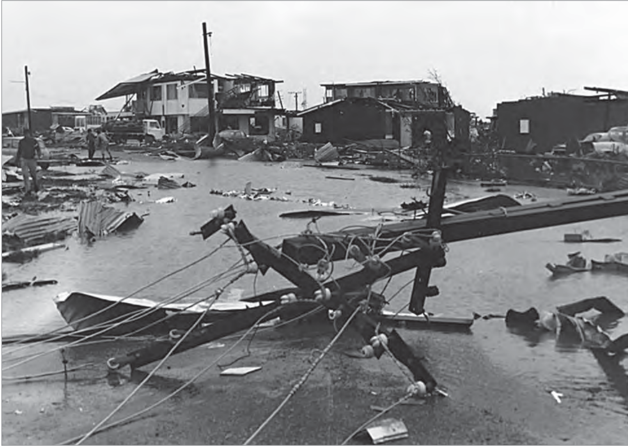
Figure A8-1 – Cyclone Tracy, Darwin, Australia, 1974 [26]
