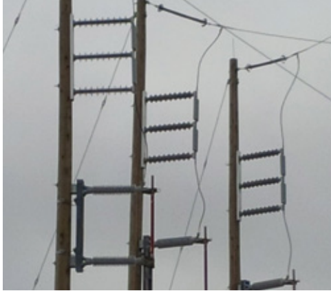
138 kV EXT current-limiting backup fuse in series with power expulsion fuse offers state-of-the-art protection. When properly coordinated, the Trans-Guard EXT current-limiting backup fuse always allows sufficient let-through current to cause the power expulsion fuse to melt and drop open, making it easy to visually pinpoint where the fault occurred.
