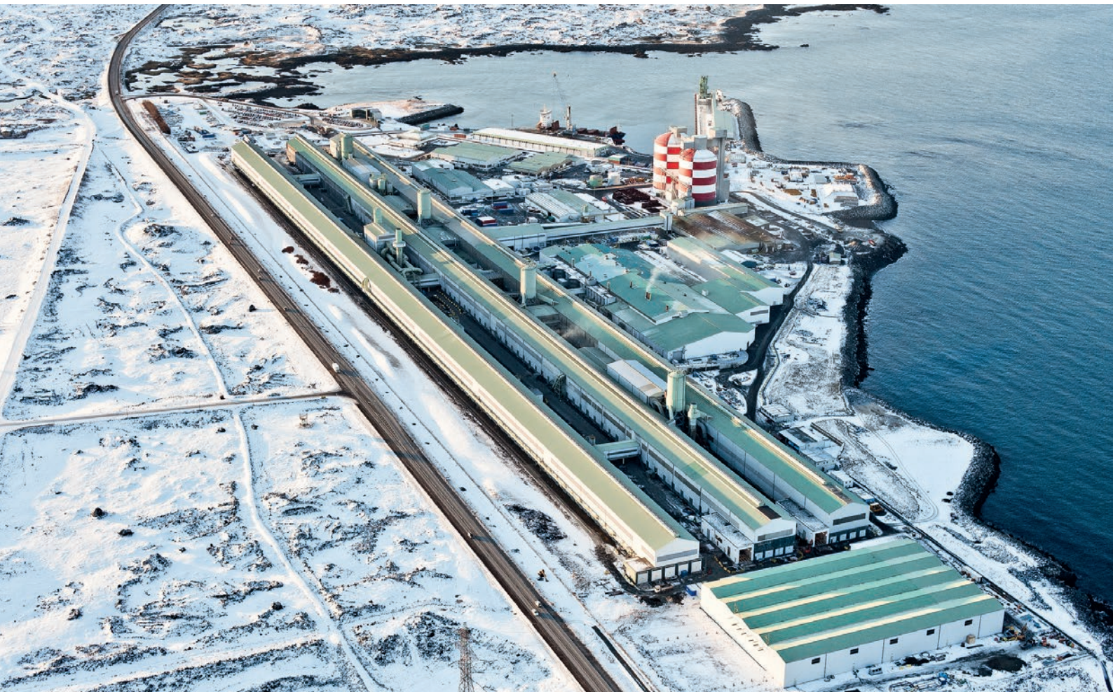
Isal aluminum plant in Iceland
