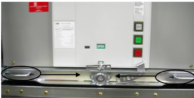
Figure 4.10 Truck handle actuation
