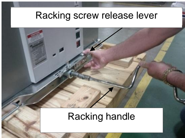
Figure 4.8 Truck racking screw
