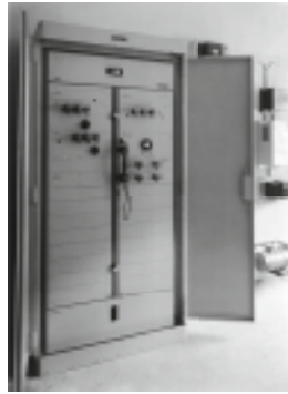
One of ABB's first utility communications installations, circa 1944. The equipment enabled grid operators to transmit signals along their own power lines.
