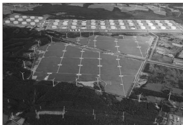
Fig.1 Panoramic view of Kamikita Rokkasho Photovoltaic Power Plant (Photo courtesy of Shin Mutsu Ogawara Inc.)
