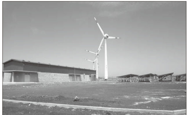
Fig.1 Panoramic view of plant
