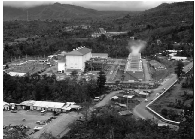
Fig.9 Panoramic view of Units 3 and 4 of Ulubelu Geothermal Power Plant
