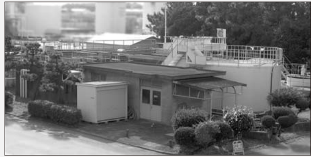
Fig.8 Wastewater treatment facility
