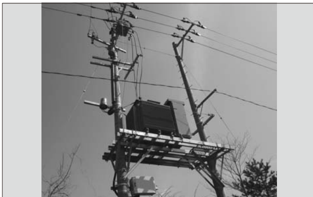
Fig.7 Variable impedance type distribution SVC in field test
